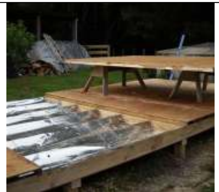
Building Panels have attractive brown building paper to walls. Natural T&G Redwood Roof & Floor supplied with Roof/ underfloor insulation paper.
